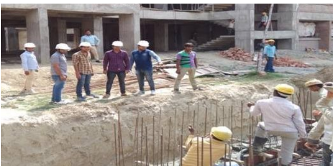
Design, Drafting and Estimation of a Hostel Building in an area of 750 Sq. Mt.
